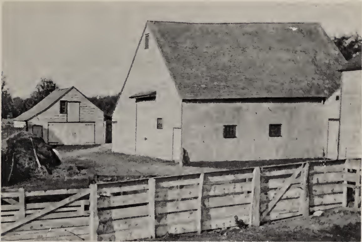
BARNYARD AT LAKE FARM with Dutch Barn (center) surrounded by the other barns shown on plan in Chap. 24.
